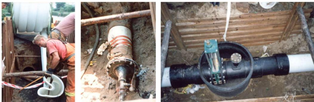
**Pictures of the Installation:** C-shape and Close-fit Installation, connected with Wavin Tegra 1000
