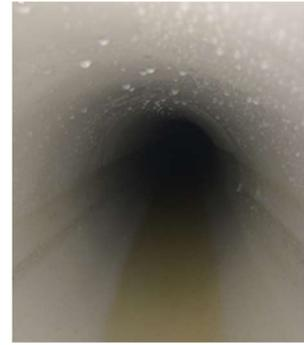
**Installation without excavation works, DN 200, SDR 26 (photos/ job supervision by Frans Alferink, Wavin Netherlands)**
